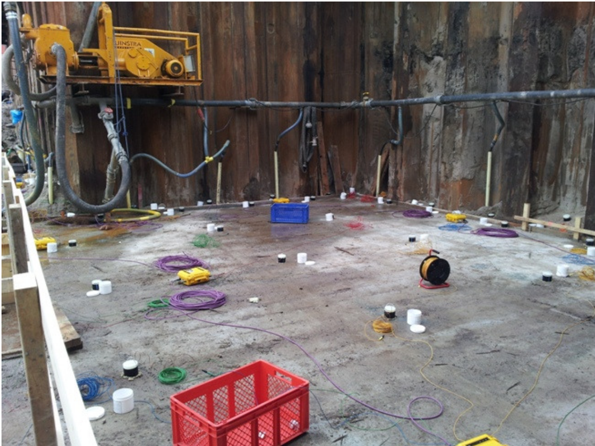
Figure 7.2. Measurement equipment installed at the building site.
