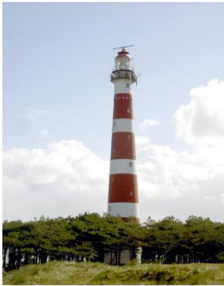
Figure 4.3. Radar on top of Ameland lighthouse (Wikipedia).
