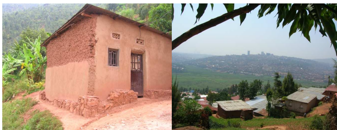
Figure 5.3: House in Nyamabuye (left), sight at centre of Kigali from Nyamabuye (right)
