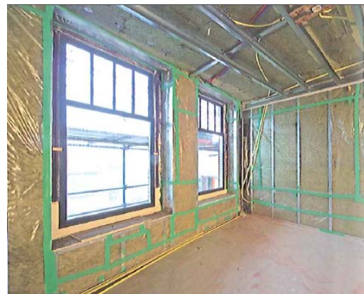
figure 3.6.6 inside insulation with taped up seams (Woonstad Rotterdam, 2011)
