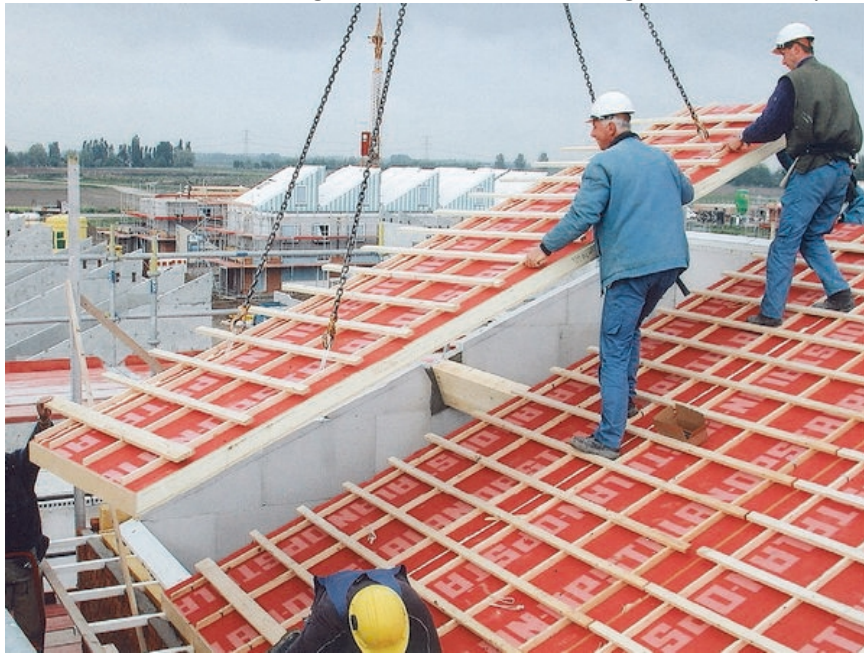
Figure 9, mounting of an insulated roof panel with tile laths (NBD, 2010)
