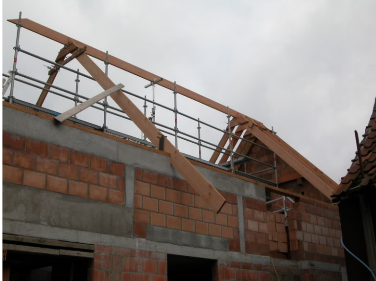
Figure 10, construction of a rafter roof (Bouwinfo, 2008a)
