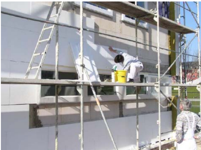
figure 6.2.7 application of VIP on a dwelling (IWU, 2009)
