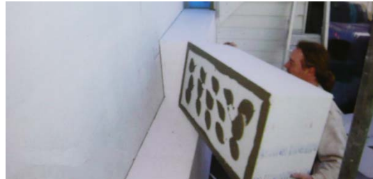
figure 3.6.7 mounting of EPS block to existing wall (Woonstad Rotterdam, 2011)
