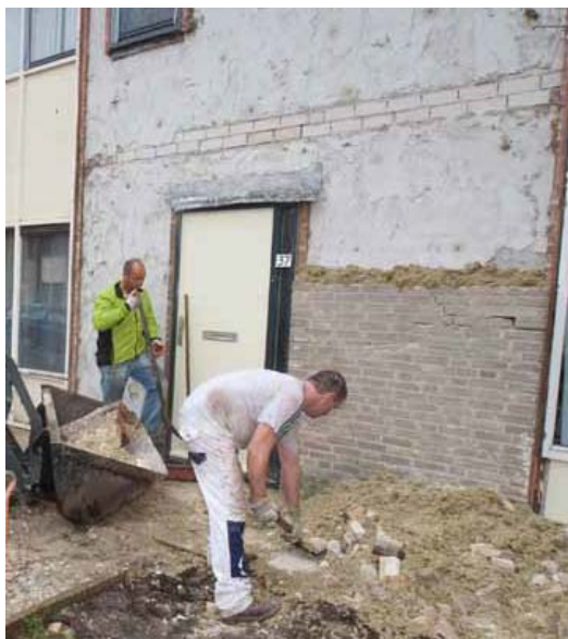
figure 3.6.3 removing the outer wall (Stichting PassiefHuis Holland, 2011)
