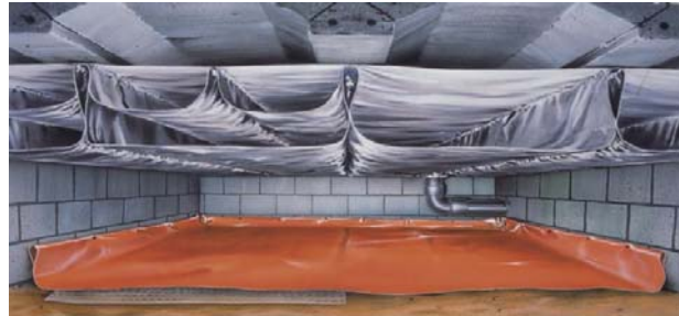
figure 6.1.1 thermosheets underneath a concrete floor (Tonzon, 2011a)
