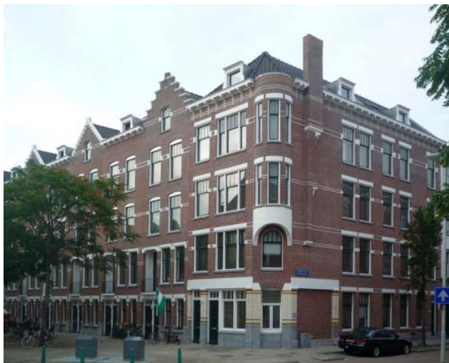
figure 3.6.8 front facade after renovation (VILLANOVA, 2009)
