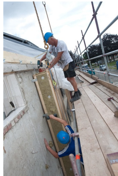
figure 3.6.4 fixing the wood timber frame elements (VDM, 2011)
