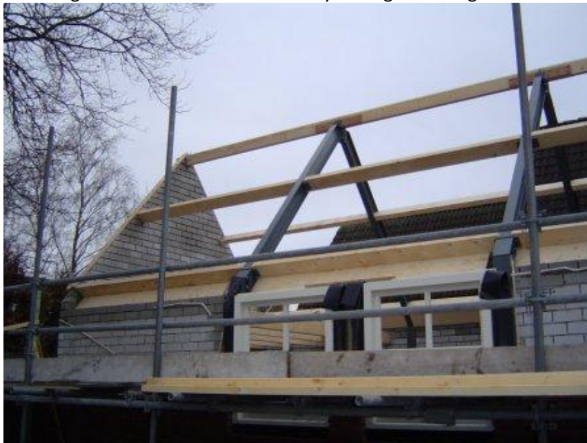
Figure 8, example of a purlin roof (Adviesbureau Simons, 2009)
