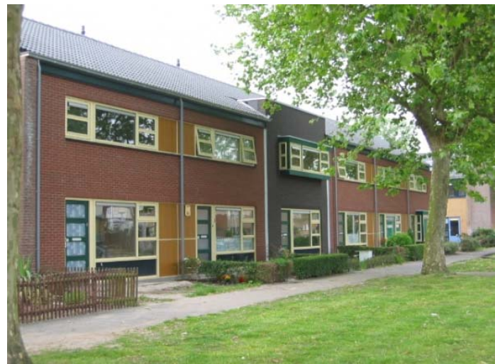
Figure 5 finished result with stone strips (Habavo, 2011)
