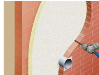
figure 4.1.6 UF-foam injected into cavity wall (Br-architect, 2010)
