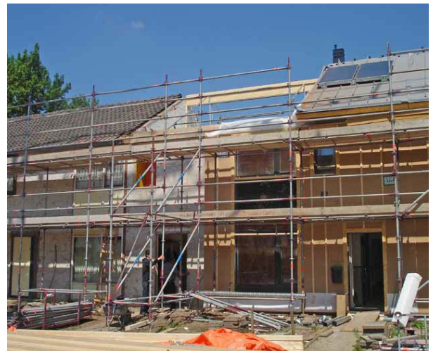
figure 3.6.1 roof placement on a terraced house in district ‘De Kroeven’ in Roosendaal (Brink Climate Systems, 2011)
