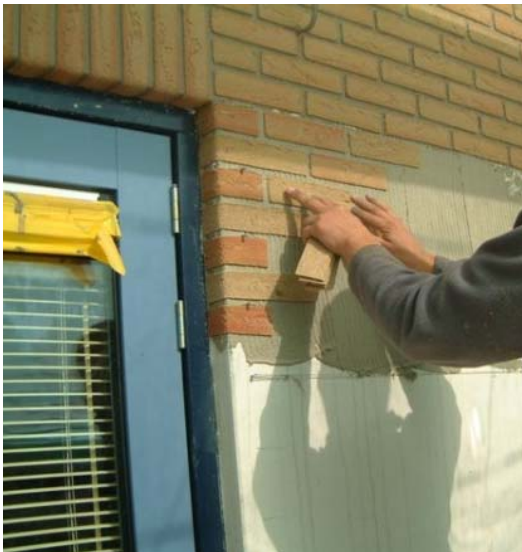
Figure 4 fixing the stone strips (Habavo, 2011)
