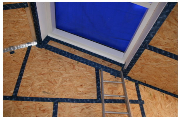
figure 3.4.2 sealing joints with tape (DWA, 2009)
