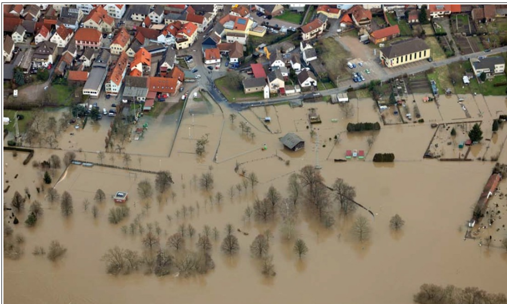
A flooded residential area (source: BMU, 2011, p. 60)
