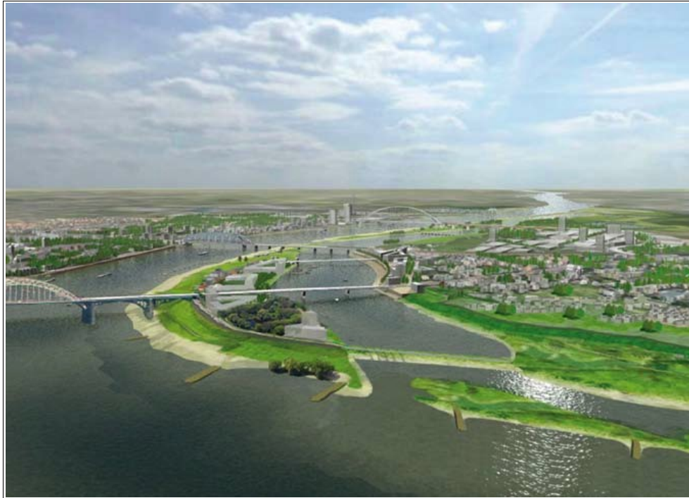
Dike relocation (artist's impression) along the Waal branch at Lent, the Netherlands
