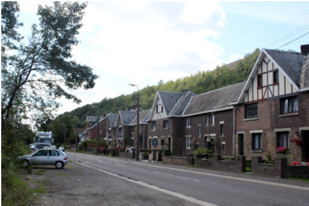
Figure 32: Rue du Fort with the basin bank on the left
