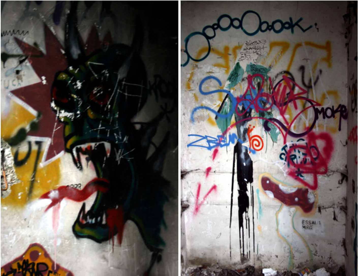
Figure 23: Examples of graffiti in the old power house
