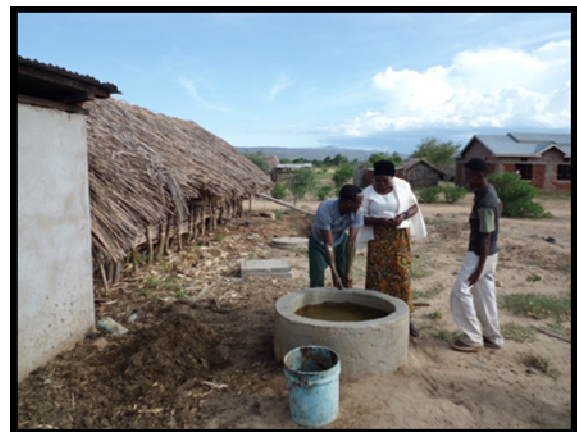
Figure 10: Mixing manure with water for the digester to operate
