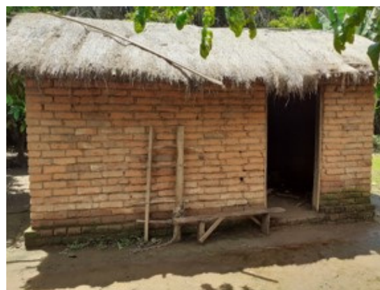
Figure 6: Semi-permanent house (MRCS, 2020)
