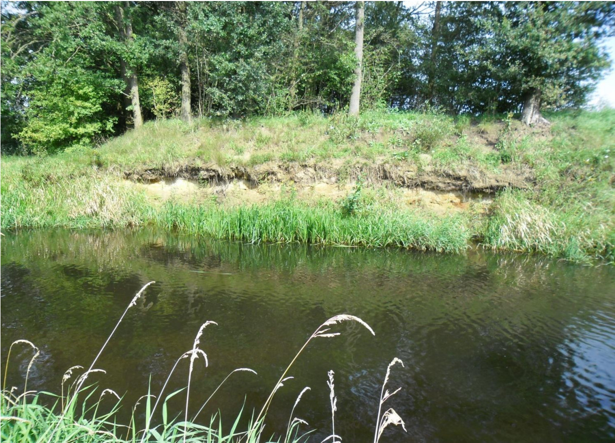
Figure 58: Erosion to the north of profile 11, east bank.
