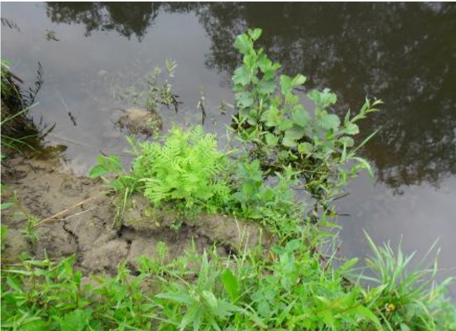
Figure 53: Active erosion at the east bank of profile 8, slides and tension cracks are visible.
