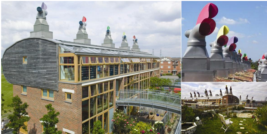
Figure 3: (Left) Beddington Zero Energy Development, Hackbridge, London. (Right) Detail of wind cowls providing passive ventilation with heat recovery (Sources: Sustainable Cities, CABE)
