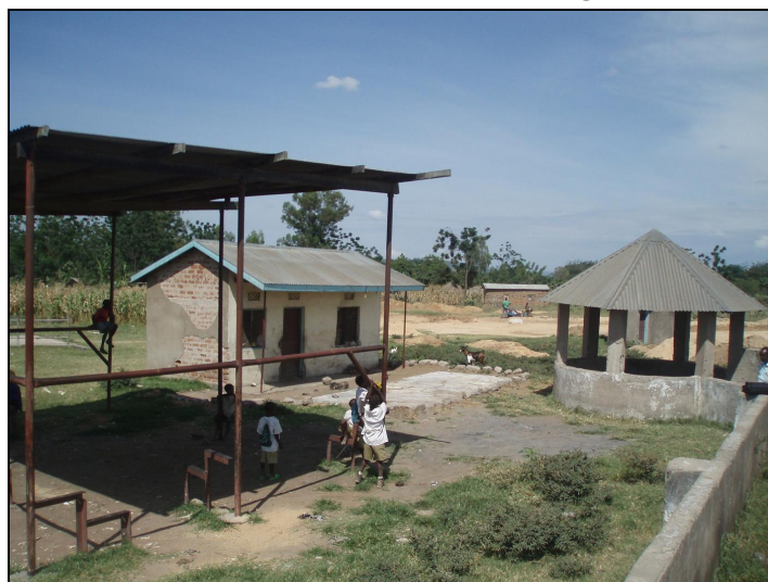
Photo 4.15 Dilapidated infrastructures, Sengerema market
