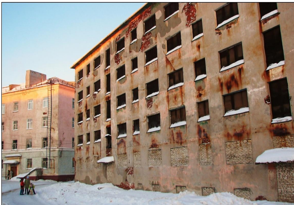
Figure 2.9 – An abandoned residential block in Kirovsk.
