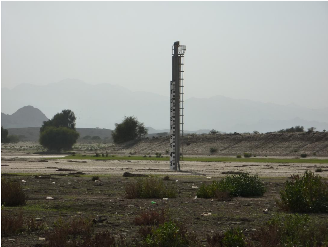
Fig. 4.1; Measuring stick behind Wadi Al-Jizi dam used to measure water levels retained by the dam after precipitation. Notice how the soil starts at 2,5 m rather than 0 meters.
