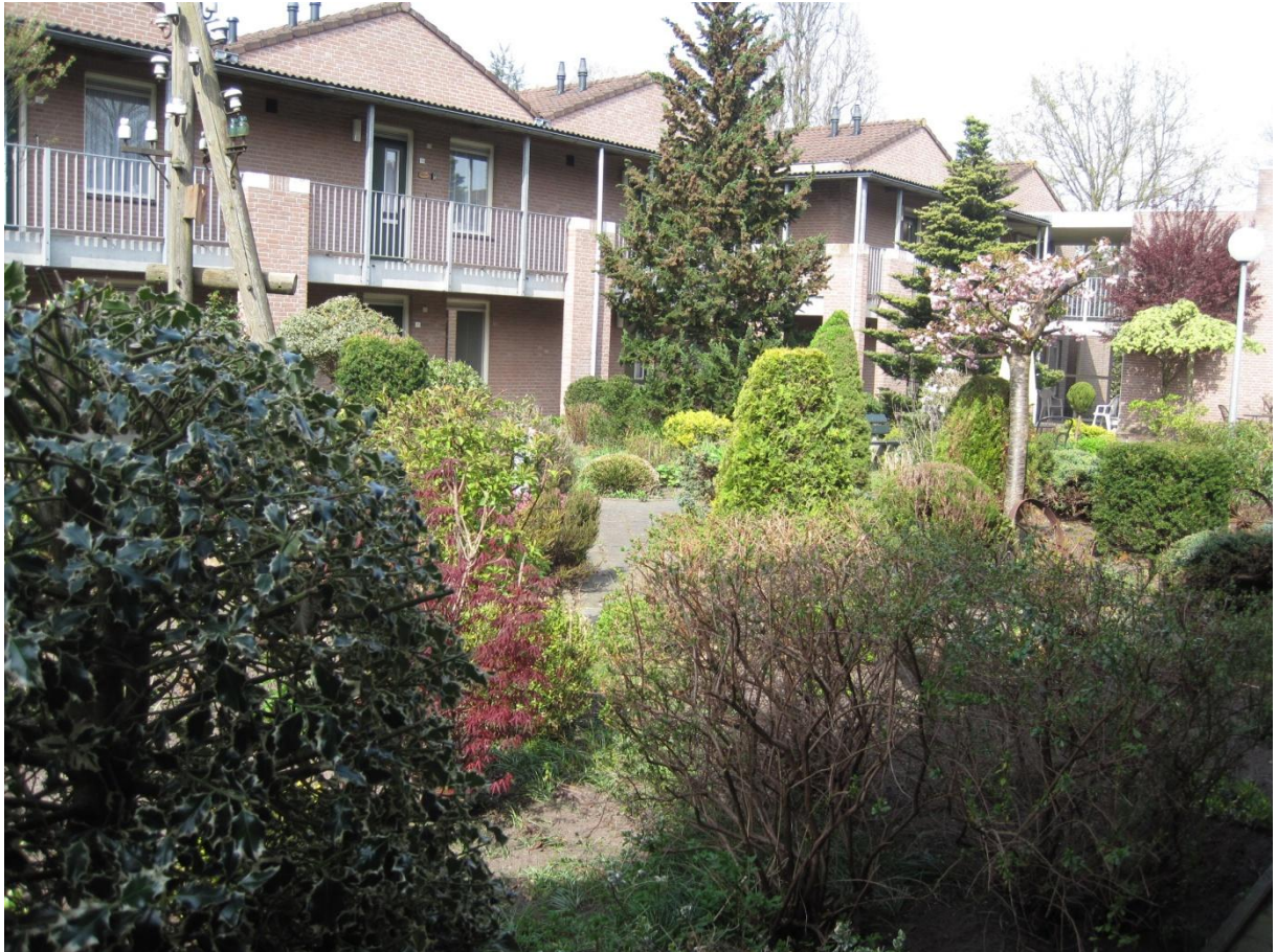
Inner garden in a residential care facility 1
